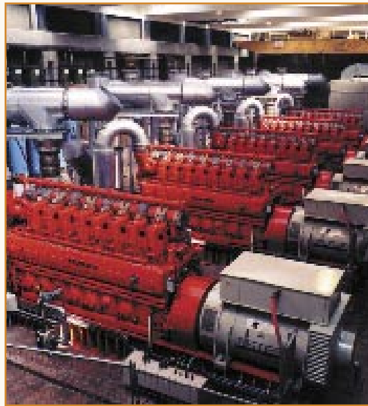
Rugged, affordable reciprocating engines can be used in industrial, commercial, institutional, and residential applications.
